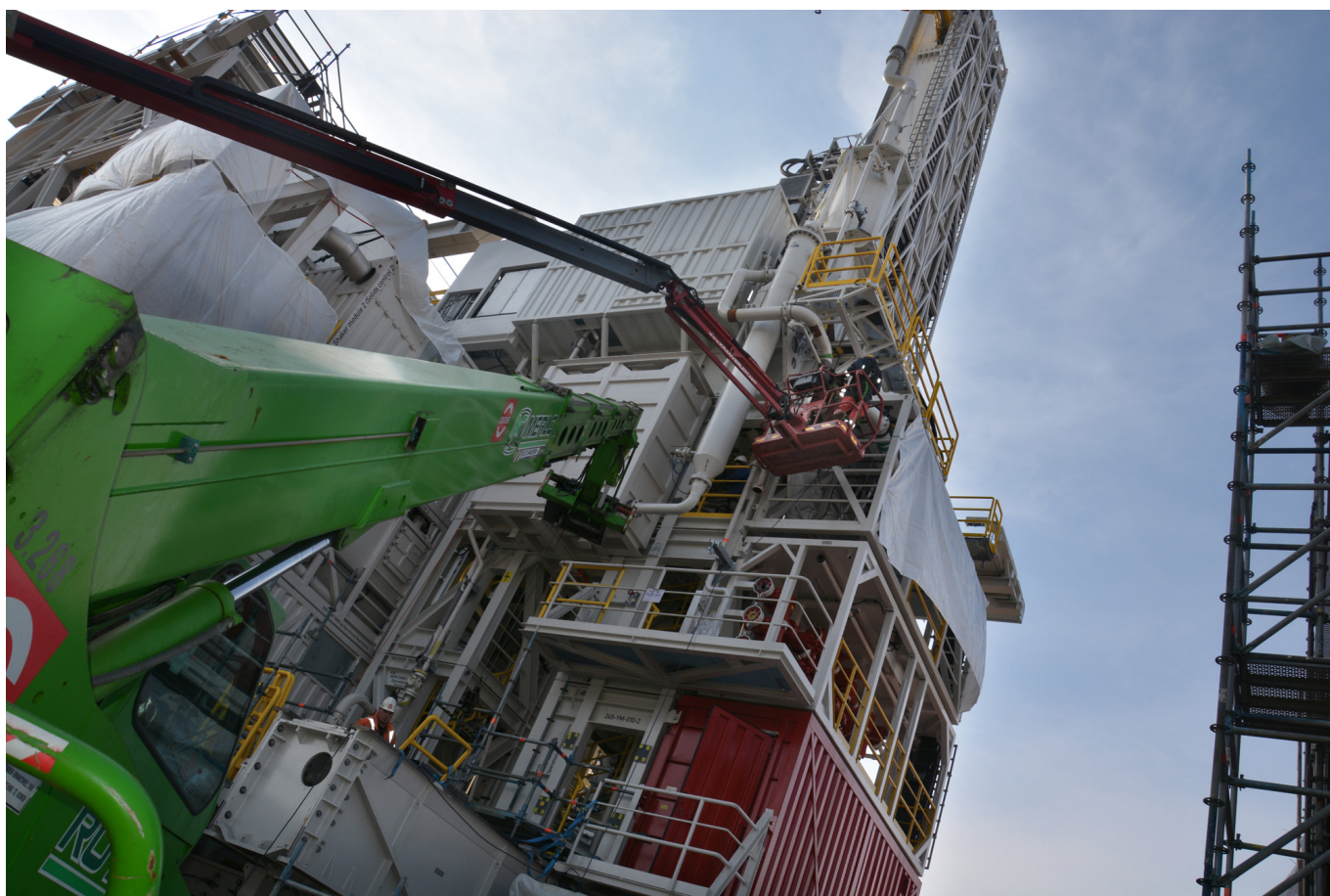
Fig. 4: Installation work on the VDD 400.2 offshore deep drilling rig (photo: Jacob)
