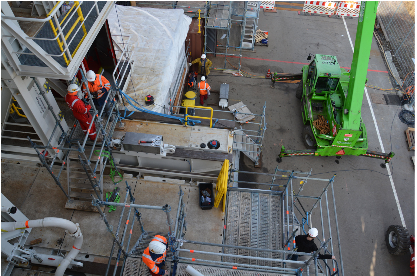
Fig. 5: Installation work on the VDD 400.2 offshore deep drilling rig (photo: Jacob)
